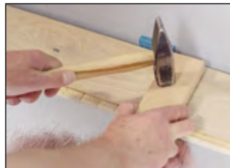
Join head joints using a hammer and protective block. The long and head joints will connect automatically. Continue this installation throughout the whole room.
