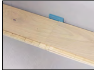
Use the plastic spacers to maintain a clearance of at least 10 to 15 mm from all walls and fixed objects in the room..
