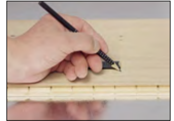
Cut the last plank of the first row to the necessary length, considering the wall clearance. The cut piece of the plank is used to start the second row.
