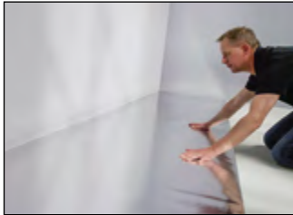
Lay out the underlay on the prepared substrate.
